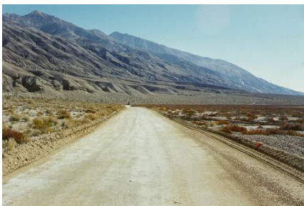
... to a mining haul road ...
