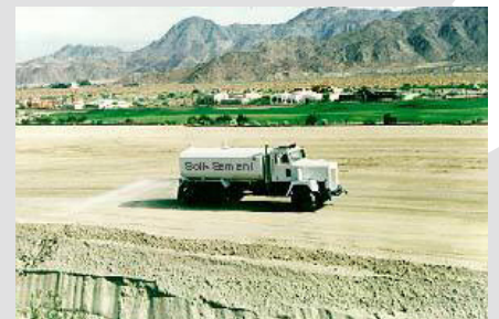
Soil-Sement® applied to a construction site ...
